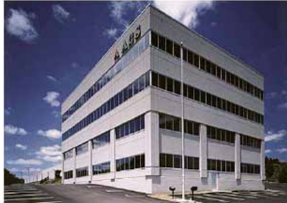
Exhibit 10-22. ACS' Pittsburgh Data Center This center houses the equipment, systems, and personnel necessary to provide world-class quality and cost-efficient services.
